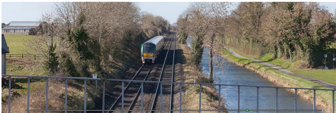
Figure 5.1 View from Pike Bridge to the Proposed New Bridge on the Eastern Ring Road
